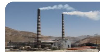
Smelter Plants (Cu Anode & Sulfuric Acid)
