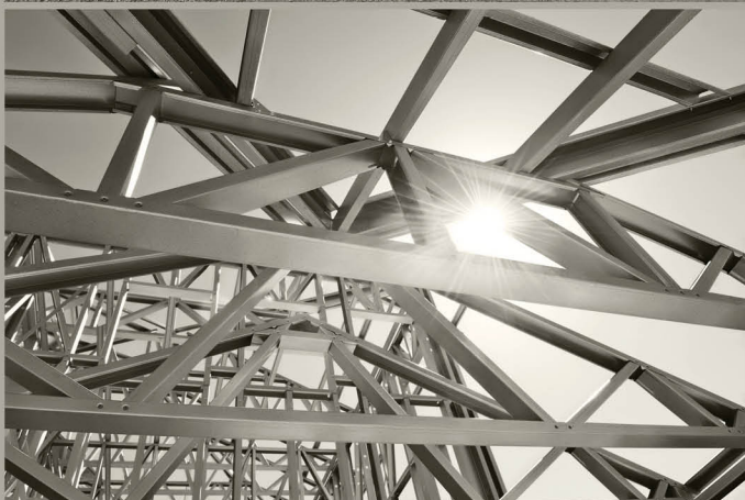
Steel Structures & Plate Works Fabrications
