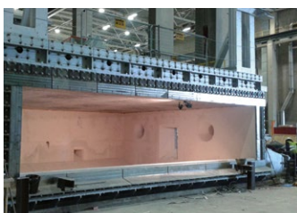
\ Complete reverberatory furnace lining in refractory concrete
